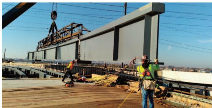
On Interstate 95 in southeastern Pennsylvania, we are constructing the first curved steel tubular flange girder bridge in the United States. The use of a tubular flange in place of a standard plate increases structural performance while reducing fabrication and erection material, as well as erection time compared to standard plate flange curved girders.
