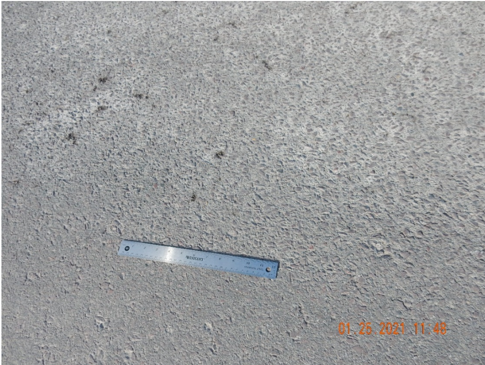
Figure 7. Closeup of the segregation mat on the eastbound lane of SR 1016 – View 1
