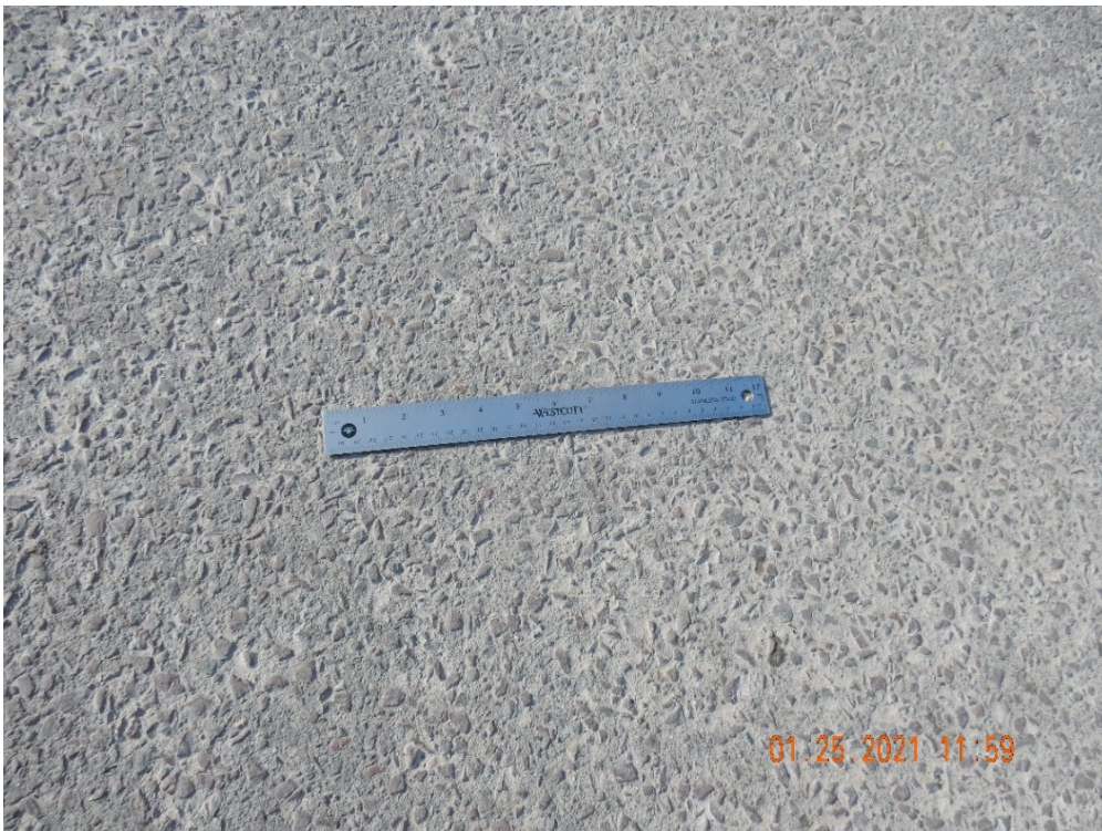
Figure 8. Closeup of the segregated mat on the eastbound lane of SR 1016 – View 2
