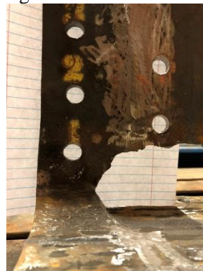
d) bearing region following testing and removal of stiffeners
