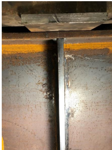
a) yield lines expressed in mill scale under point of application of load
