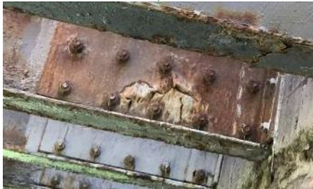
c) bolted steel 'splice' anchored to existing end diaphragm Figure 35 Repair approaches for embedded bearing regions.
