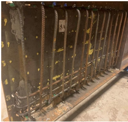
a) Girder 5A
