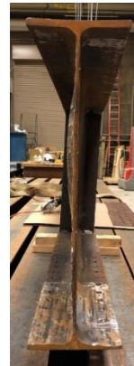
b) web distortion following testing and removal of stiffeners
