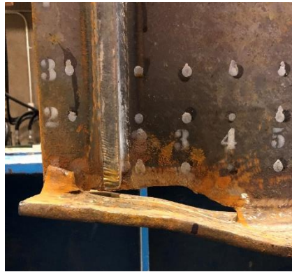
b) residual distortion of bearing region after testing
