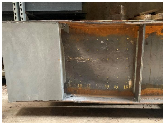
Figure 60 Girder 4B following testing showing panel buckling of the unencased portion of the web.
