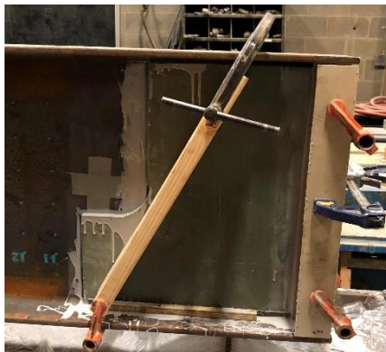
installation of FRP
