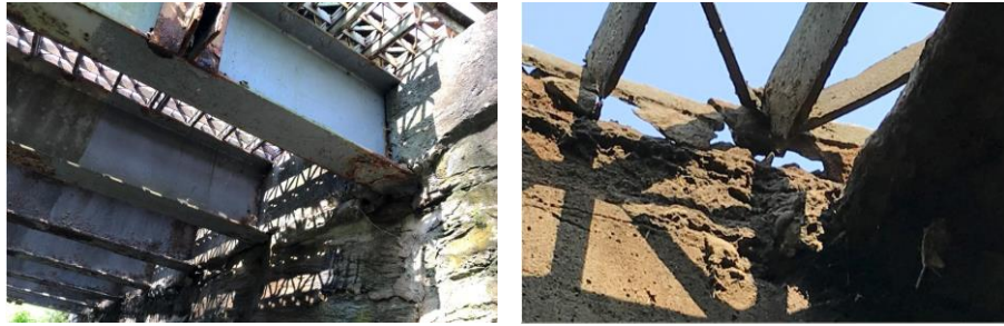
a) condition of far abutment prior to encasement (pre 2020)
