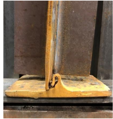
c) complete collapse of the web
