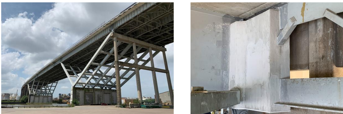
Figure 20 Field implementation of UHPC reported by TxDOT (2021)
