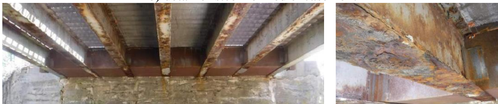
c) steel-formed concrete encasement at far abutment (post 2020)
