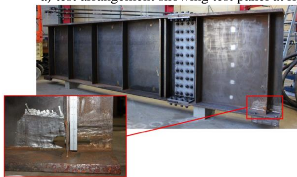
b) specimen with damaged end region
