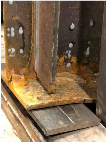
a) bearing region during testing
