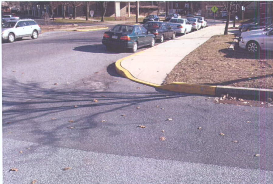
Curb cut near Middletown Station
