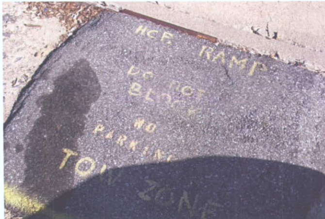
Pedestrian ramp at Lancaster Station
