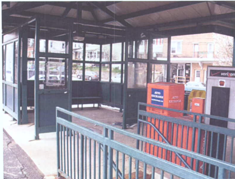
Lighting at Downingtown Station
