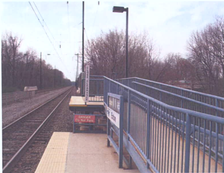
Detectable platform edge and mini-high platform at Exton Station
