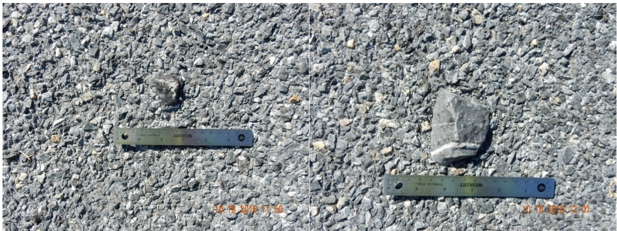
Figure 19. A few spots showed large pieces of aggregate stuck into the chip seal (southbound).
