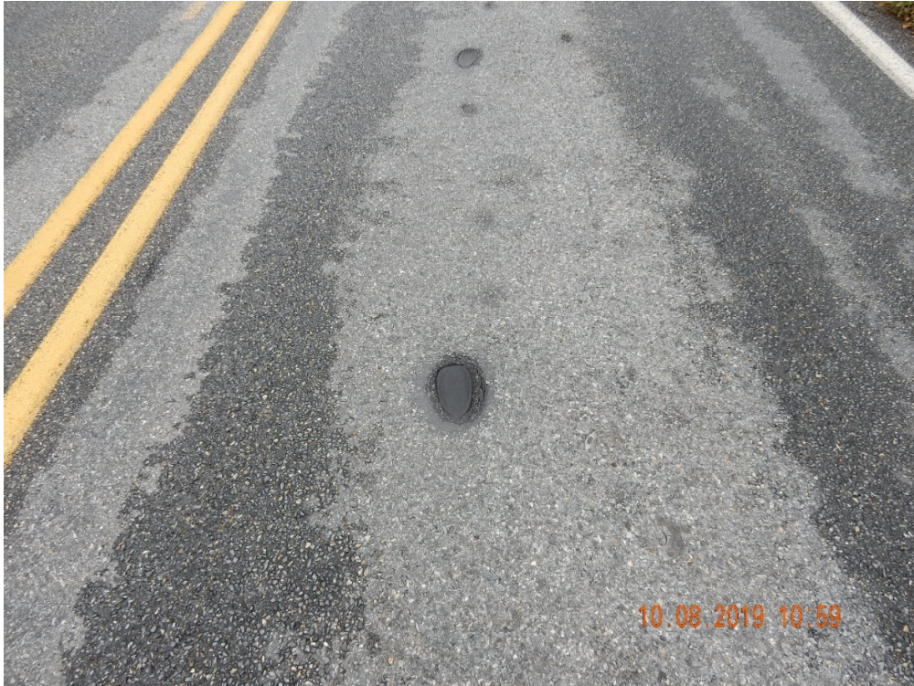
Figure 27. Spots of chip loss to the left of the mat center on the northbound.
