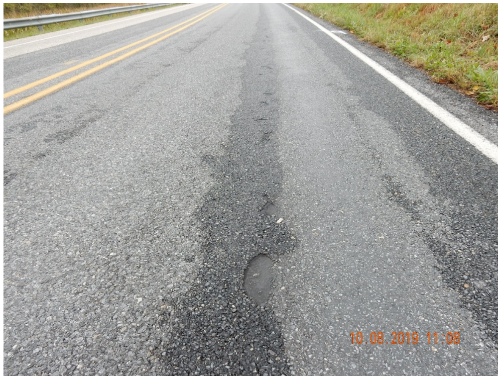
Figure 28. Spots of chip loss to the right but close to the mat center on the northbound.
