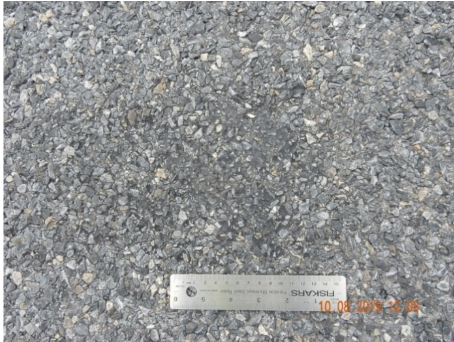
Figure 21. Overall the texture looks very good after more than a year in service.
