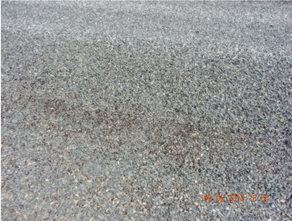
Figure 14. Finished mat after placement of the second chip seal layer.
