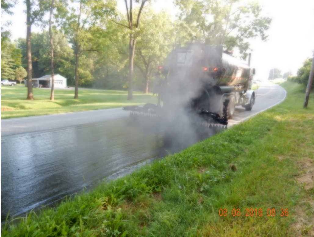
Figure 6. Placement of PG 70-22 asphalt binder on the existing pavement surface.
