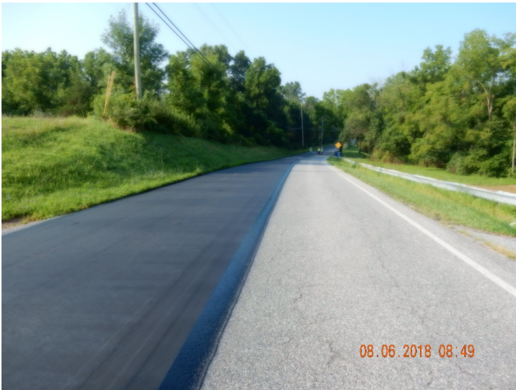
Figure 9. Geofabric placed on the tack asphalt on the northbound.
