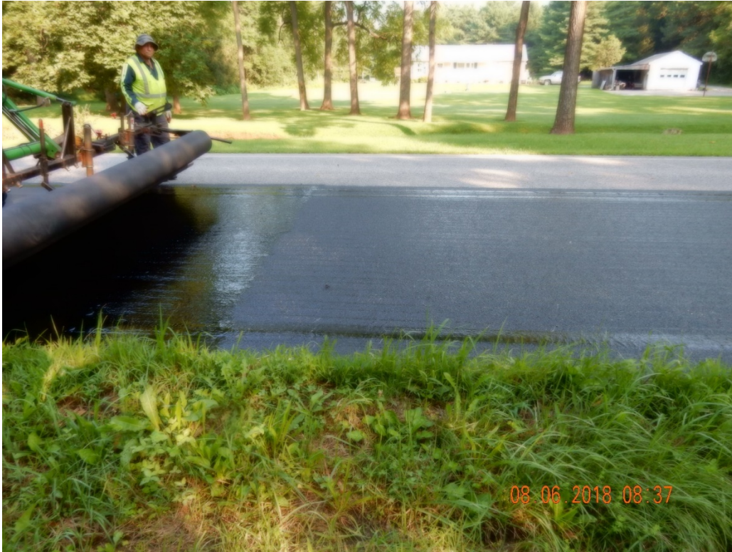
Figure 8. Placement of geofabric on the freshly placed tack coat asphalt.
