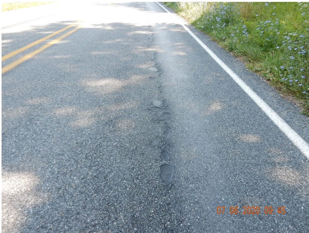
Figure 34. The chip loss spots forming an almost straight line can be seen to the right of the center on the northbound.
