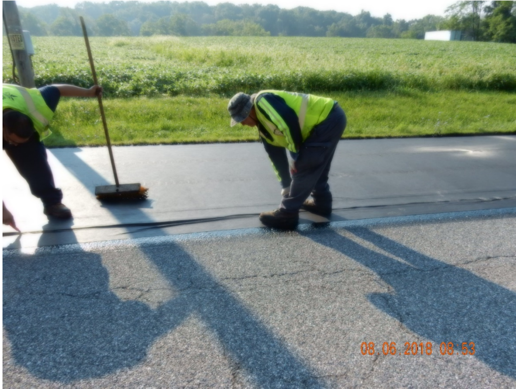
Figure 10. Cutting through wrinkled section of the geofabric to smooth it out.
