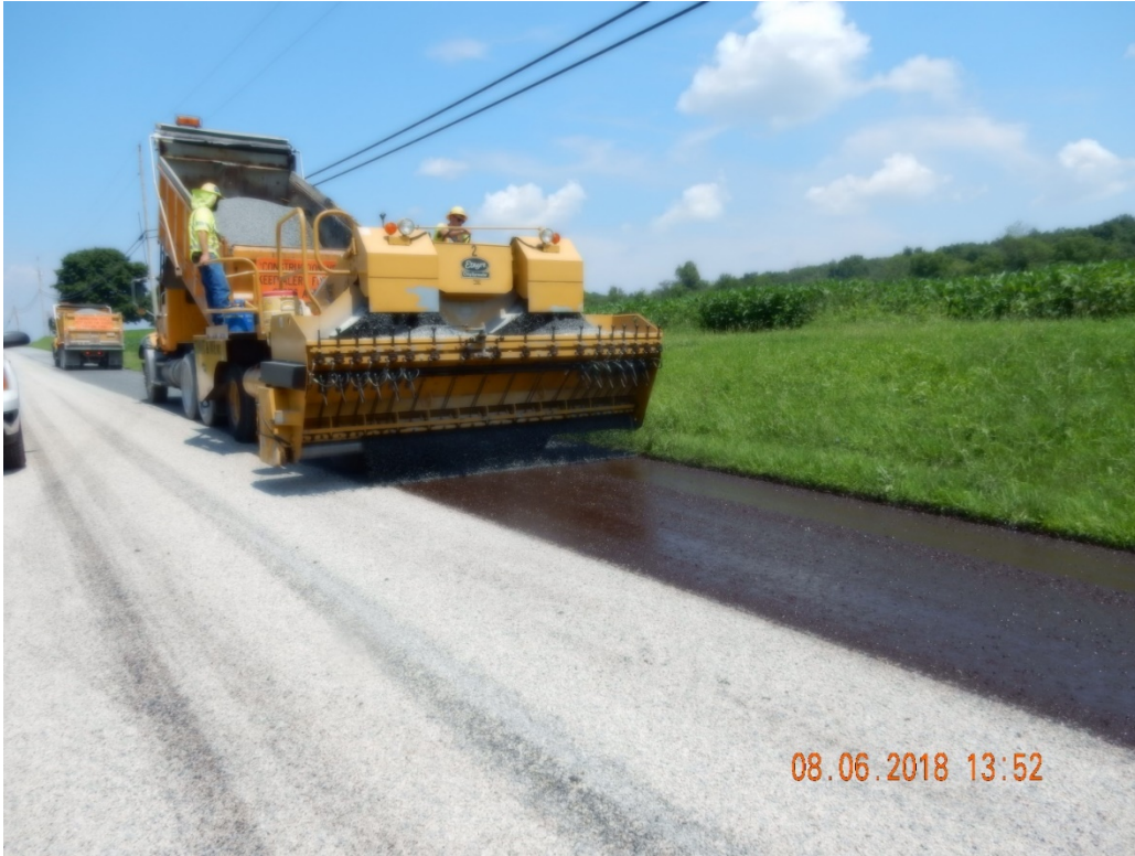
Figure 12. Spreading the #8 chips on the emulsion.
