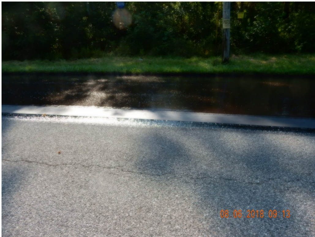
Figure 11. CRS-2P emulsion placed over geofabric before chip application.
