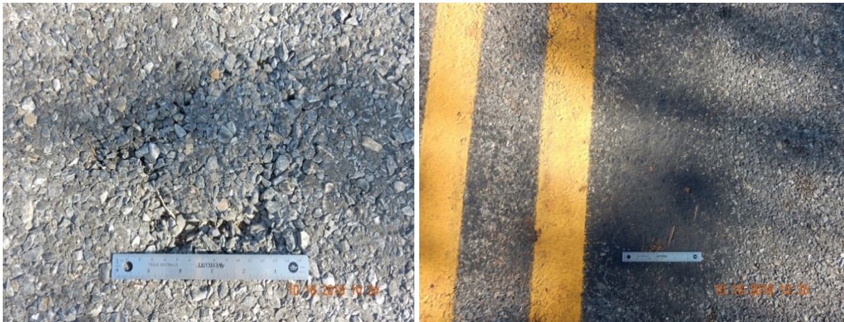
Figure 18. Several spots indicated the beginning of surface chip loss or minor bleeding.
