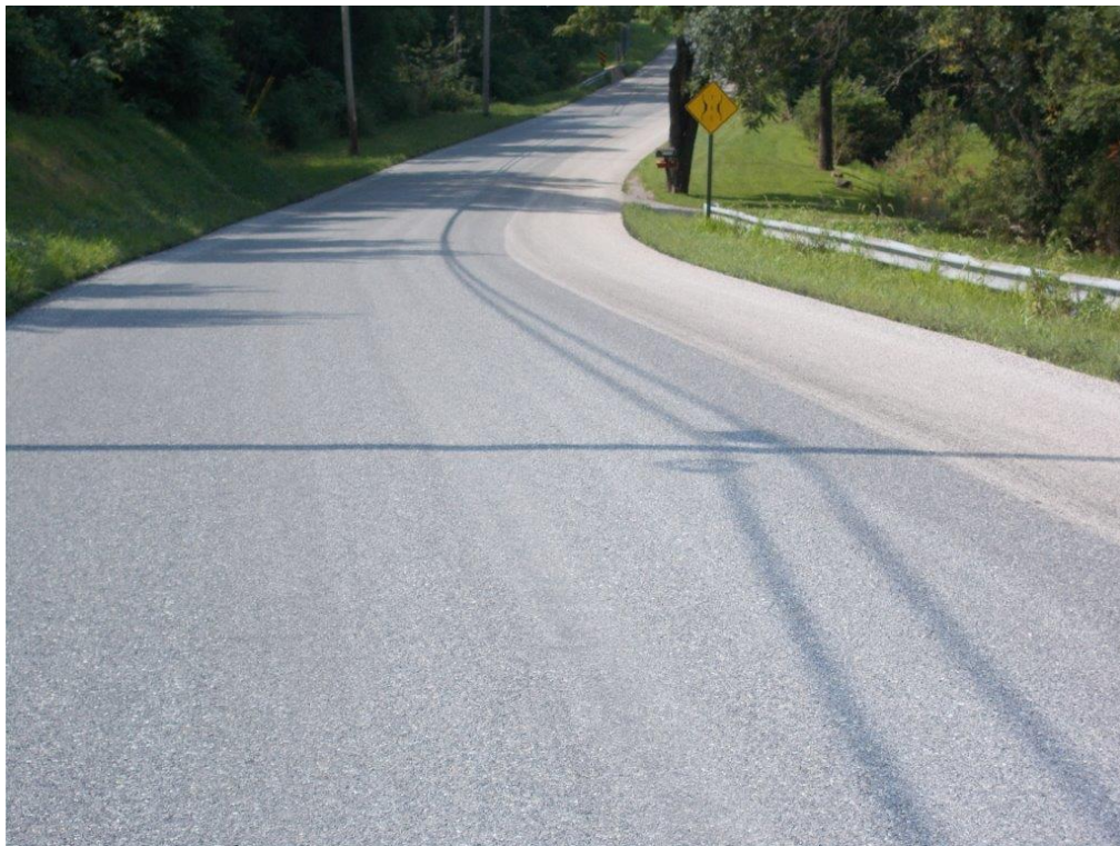
Figure 15. General appearance of the mat after 8 days in service, looking southbound.
