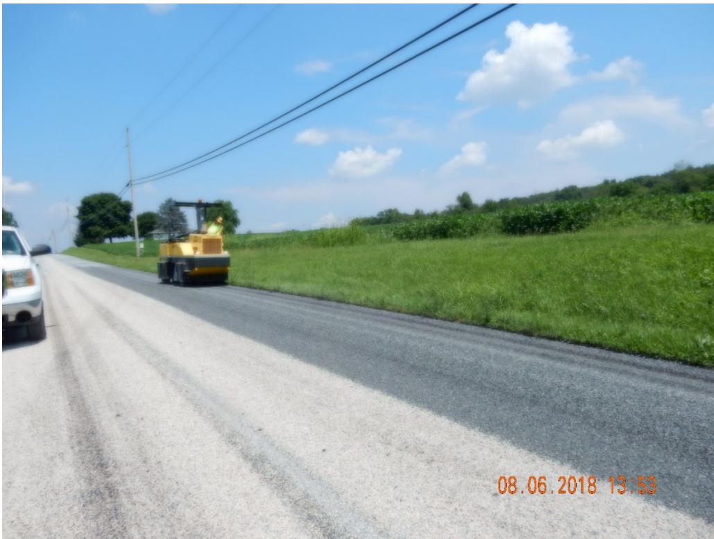
Figure 13. Rolling the second chip seal layer.
