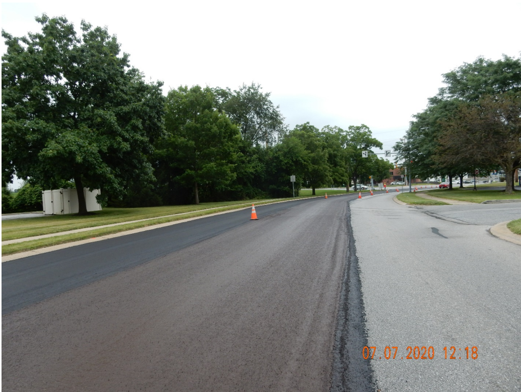
Figure 13. Freshly placed micro on the center lane.
