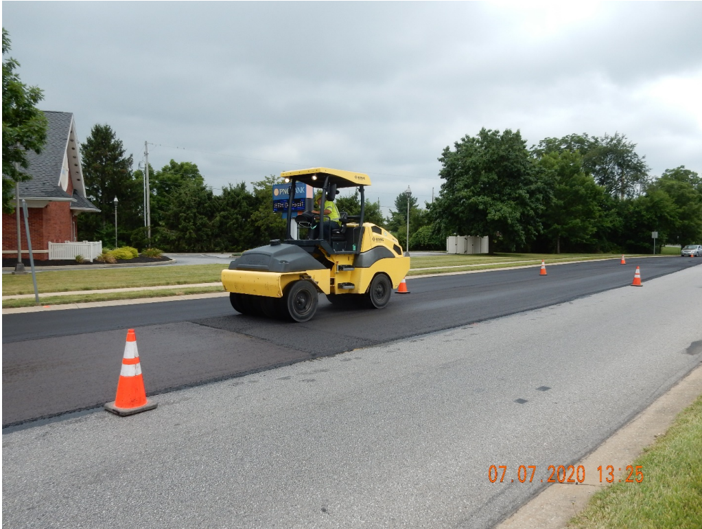
Figure 14. Compacting the center lane micro (second layer).
