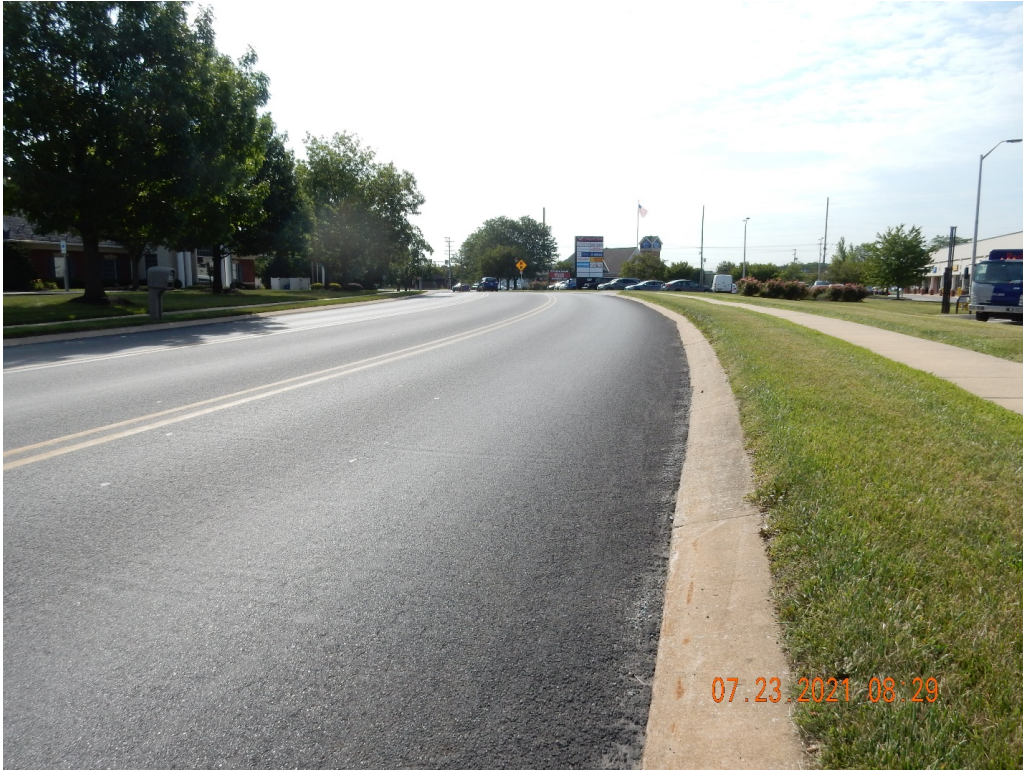
Figure 17. A general view of the micro after one year in service, looking southbound.
