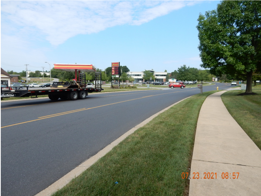
Figure 21. Another view of the micro after one year of service looking northbound.
