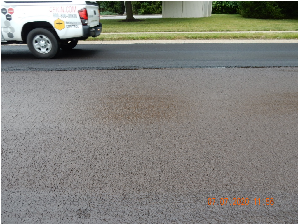
Figure 10. Cured micro on the northbound (far side) and freshly placed micro on the center lane.
