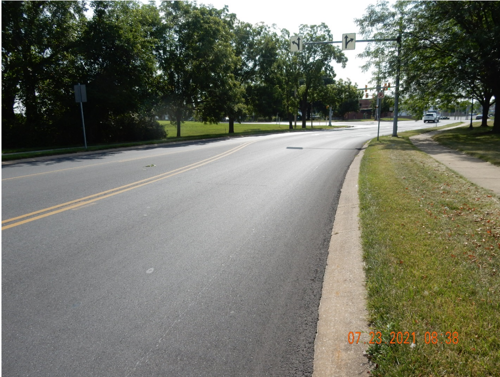
Figure 19. Excellent performance and texture after one year of service (looking southbound).
