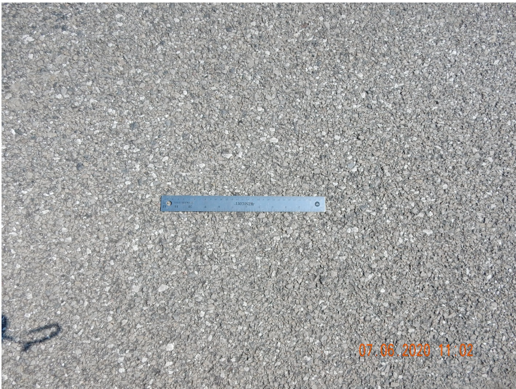
Figure 6. Close-up view of surface texture of existing pavement.
