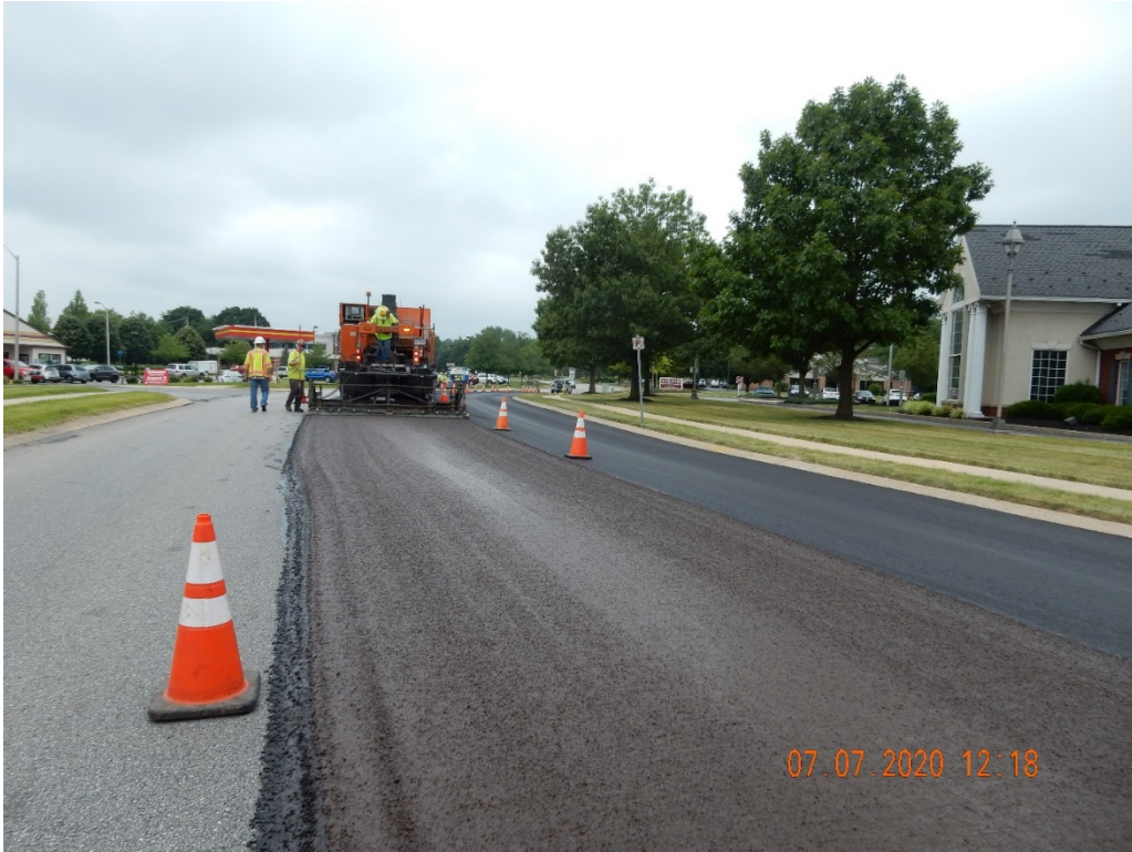
Figure 12. Placement of second layer of micro on the center lane.
