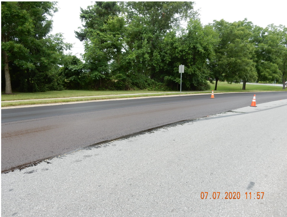
Figure 11. Completed micro (northbound), freshly placed scratch micro (center lane), and existing pavement to be paved (southbound).
