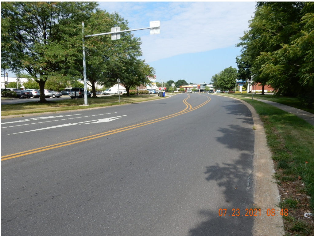
Figure 20. General view of the micro after one year of service (looking northbound).
