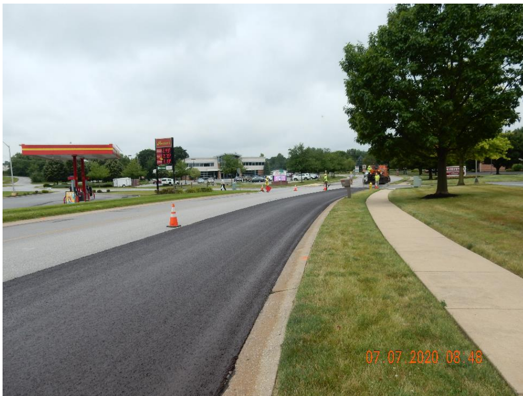
Figure 7. The scratch layer of fiber-reinforced micro surfacing placed on the northbound lane.
