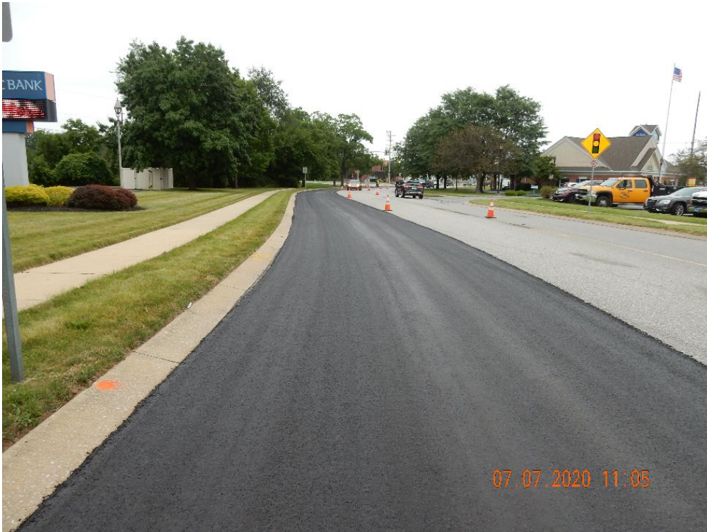
Figure 8. The top layer of fiber-reinforced micro surfacing placed on the northbound lane.
