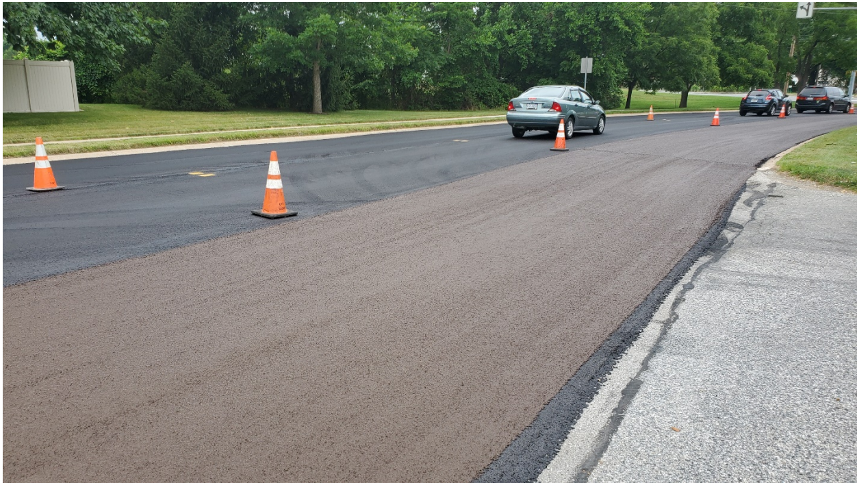
Figure 15. Completed micro on the southbound lane.
