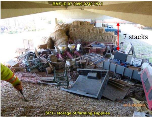
(a) Cargo stored underneath the bridge
