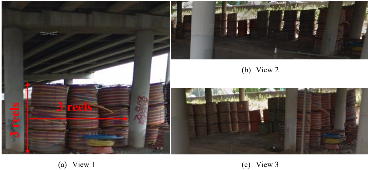
Figure 4: Views of the conduit reels stored underneath span 30NB
