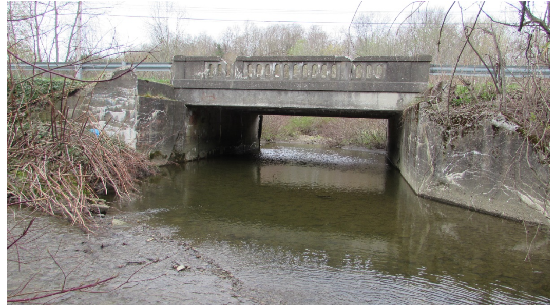
Bridge #3 over Lamson Run
