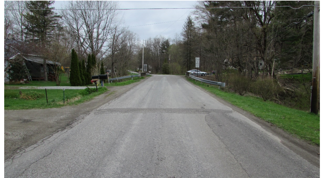
Bridge #2 Approach (Looking North)
