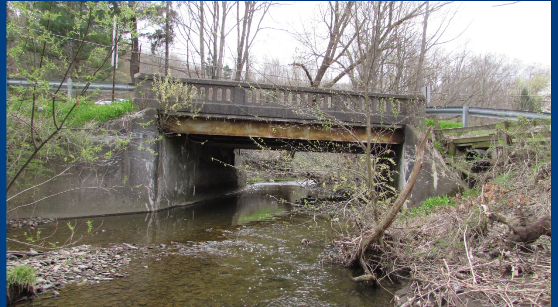
Bridge #2 over Lamson Run
