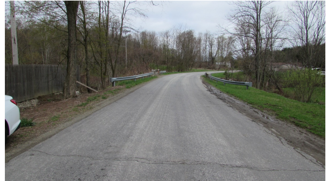
Bridge #3 Approach (Looking North)
