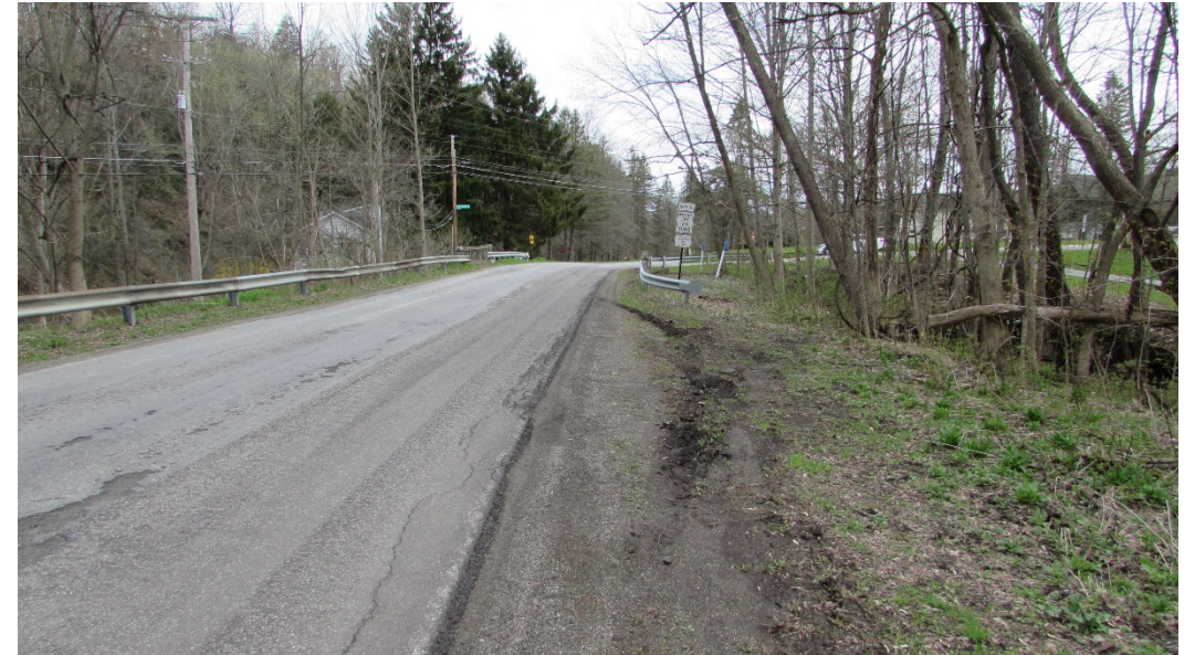
Bridge #1 Approach (Looking North)
