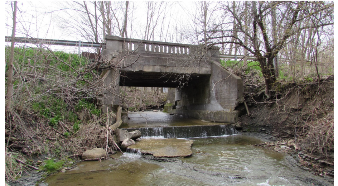
Bridge #1 over Tributary to Lamson Run
