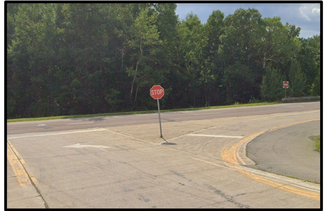
US 6 & Baldwin Park St Road Intersection
