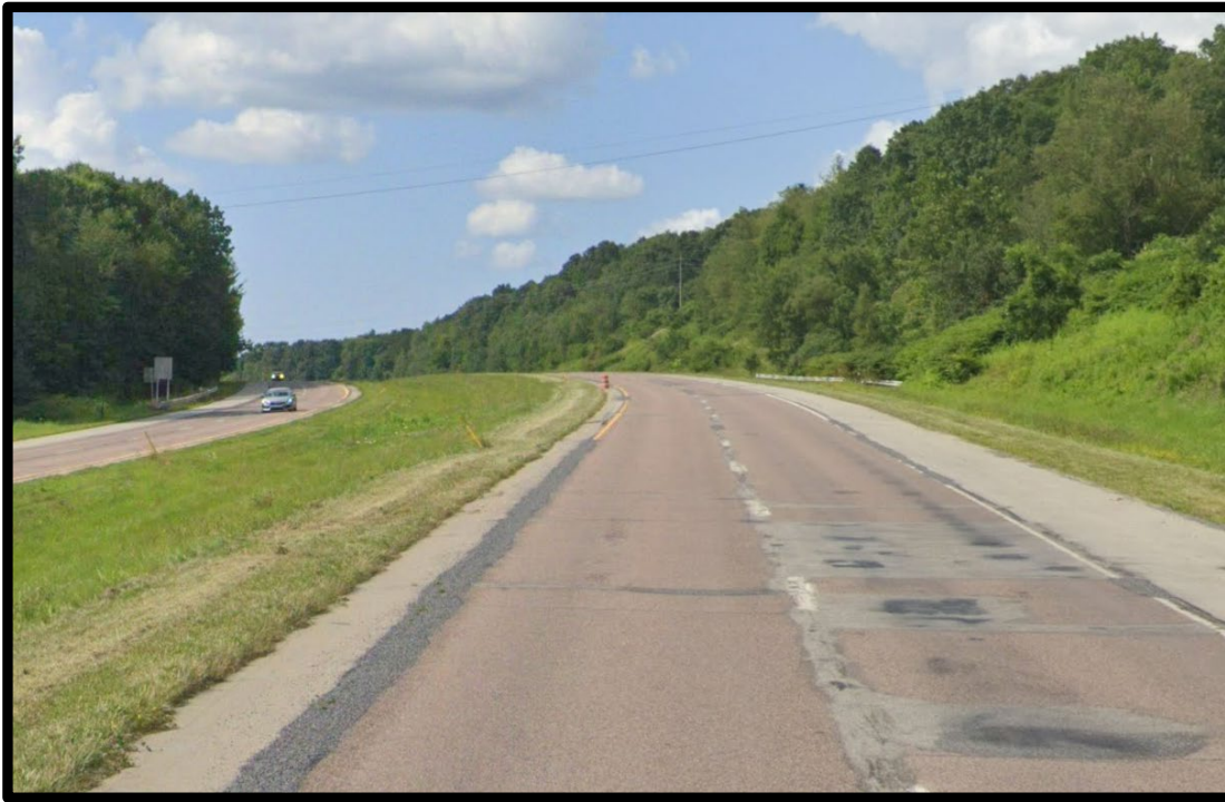
Existing US 6 Eastbound Lanes
