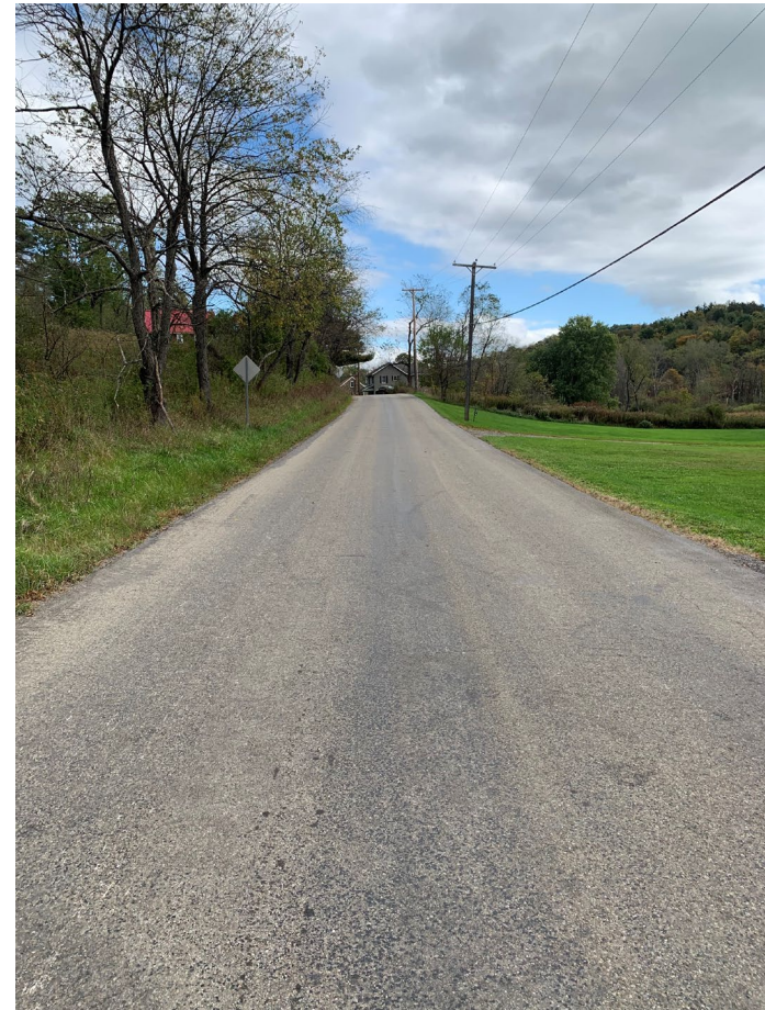
Roadway - Looking East (Towards Troutville)
