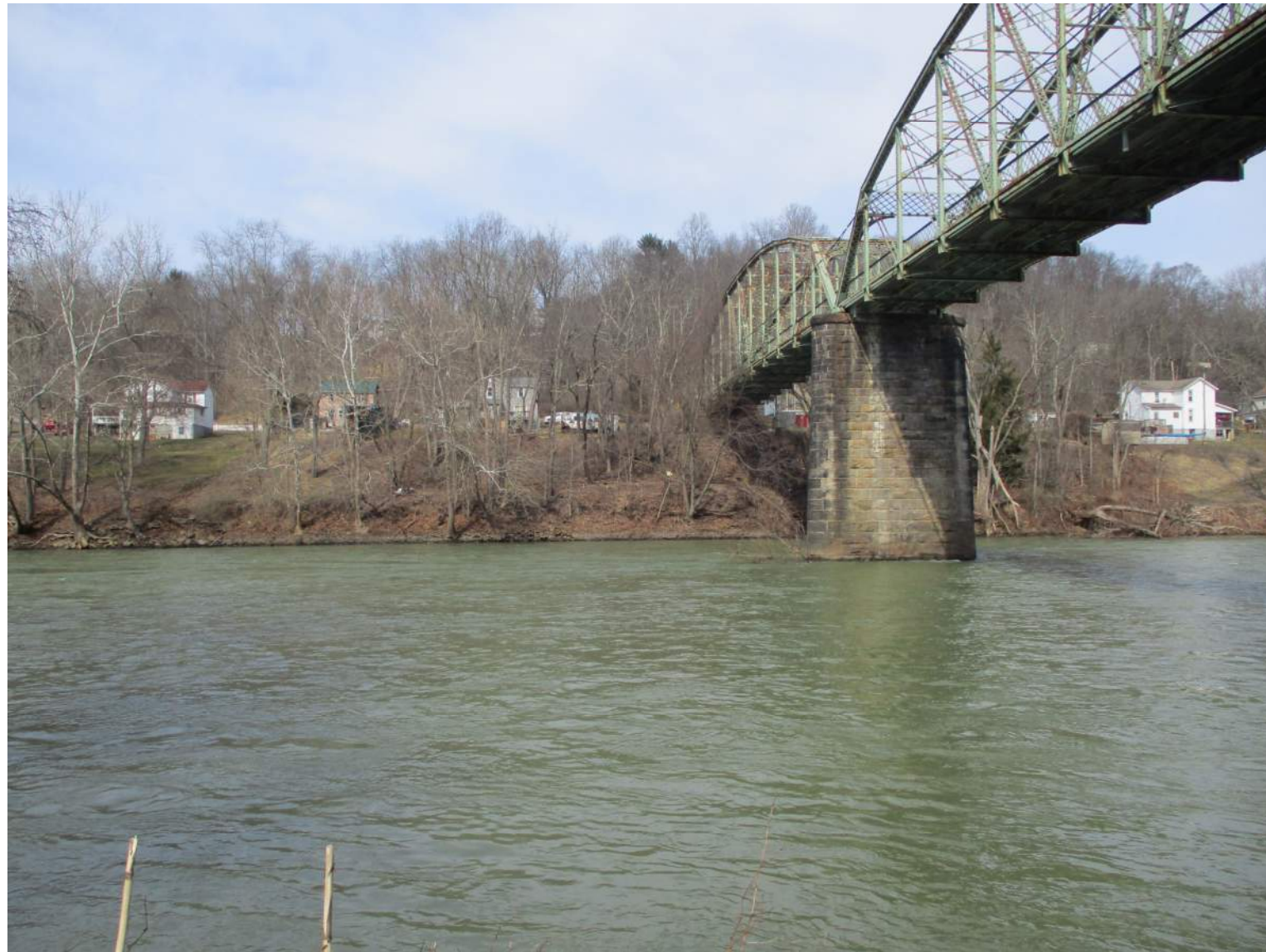
Looking towards Armstrong Co (Proposed Bridge Location)
