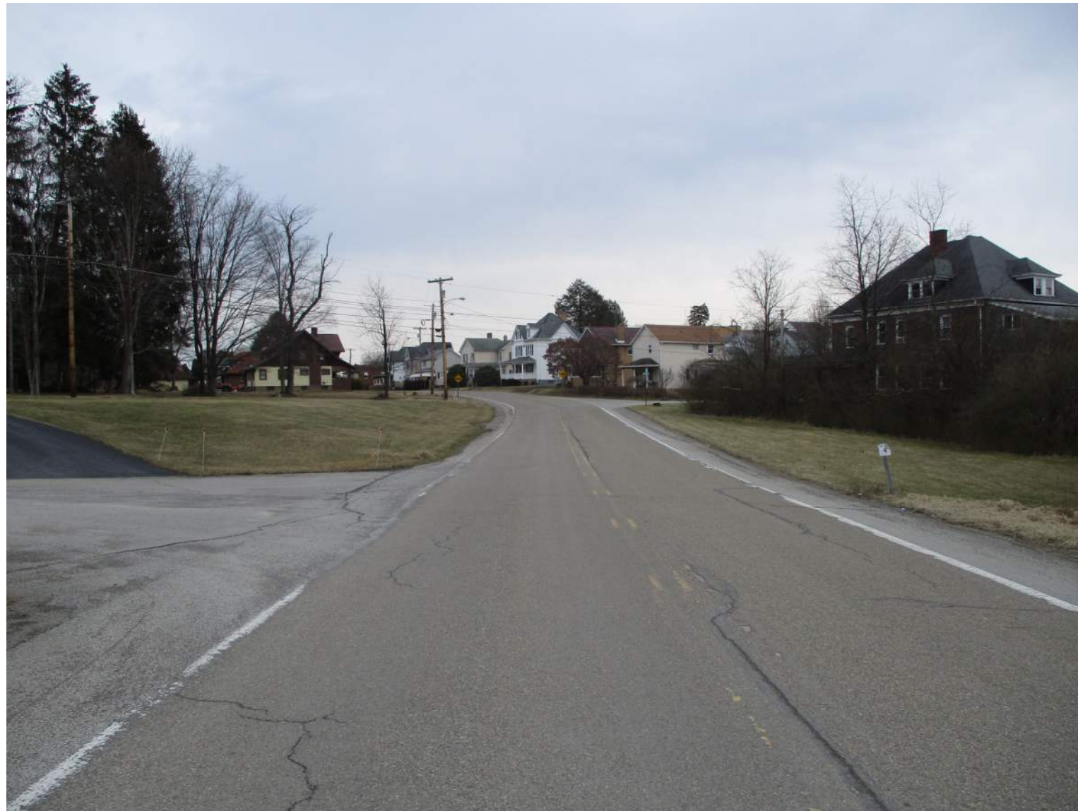
Looking East on SR 1060 (Main St) Westmoreland Co (Mill and Overlay from SR 0981 to Kier St)
