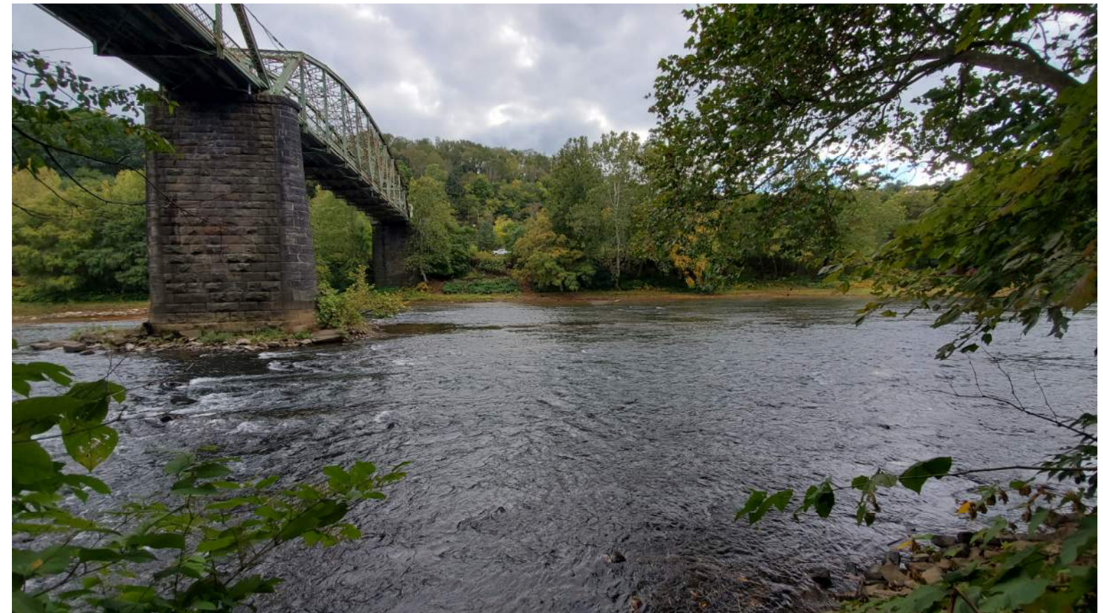
Looking towards Westmoreland Co (Proposed Bridge Location)
