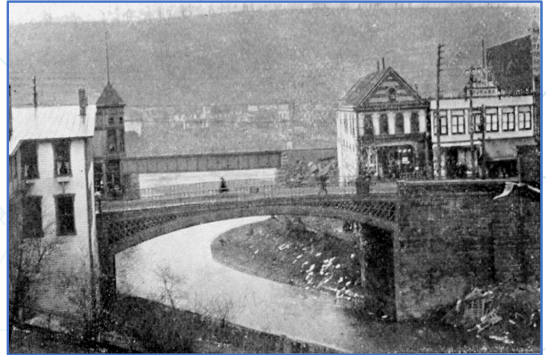
Dunlap Creek Bridge circa 1904 (right image)
