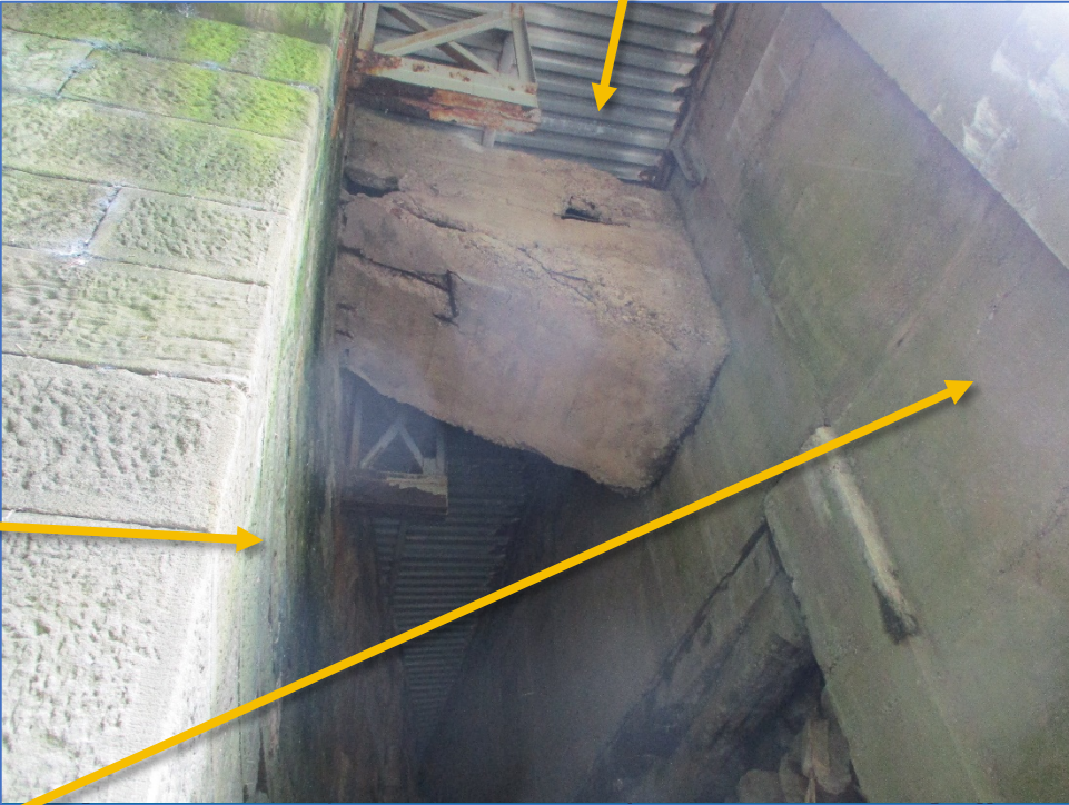
Sidewalk SIP Forms
