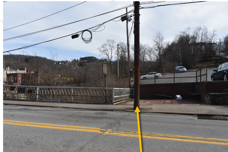
Remove Existing Steel Poles
