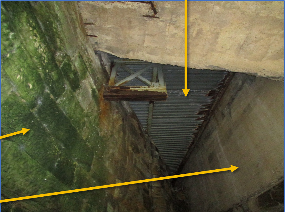
Sidewalk SIP Forms
