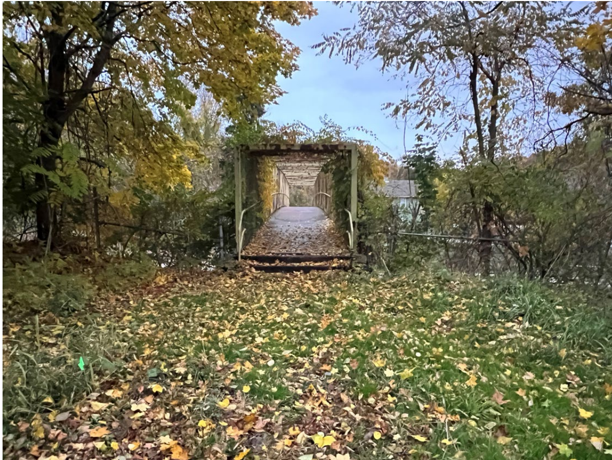
EXISTING PEDESTRIAN BRIDGE VIEW LOOKING NORTHWEST
