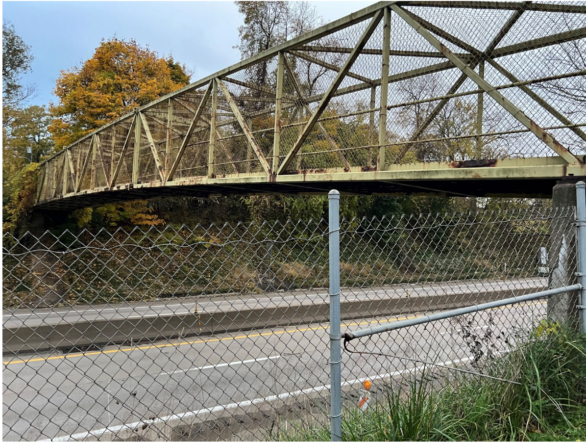
EXISTING PEDESTRIAN BRIDGE VIEW LOOKING SOUTHWEST
