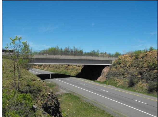
Photograph 1: Hazleton Beltway (S.R. 0424) bridge over I-81. All proposed build alternatives would extend from this location northward into HIP (June 2008).
