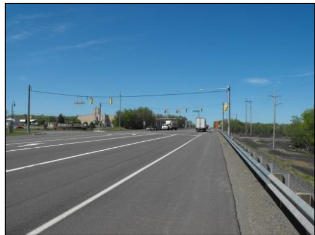
Photograph 3: Access road to Humboldt Station from S.R. 0924 (June 2016).
