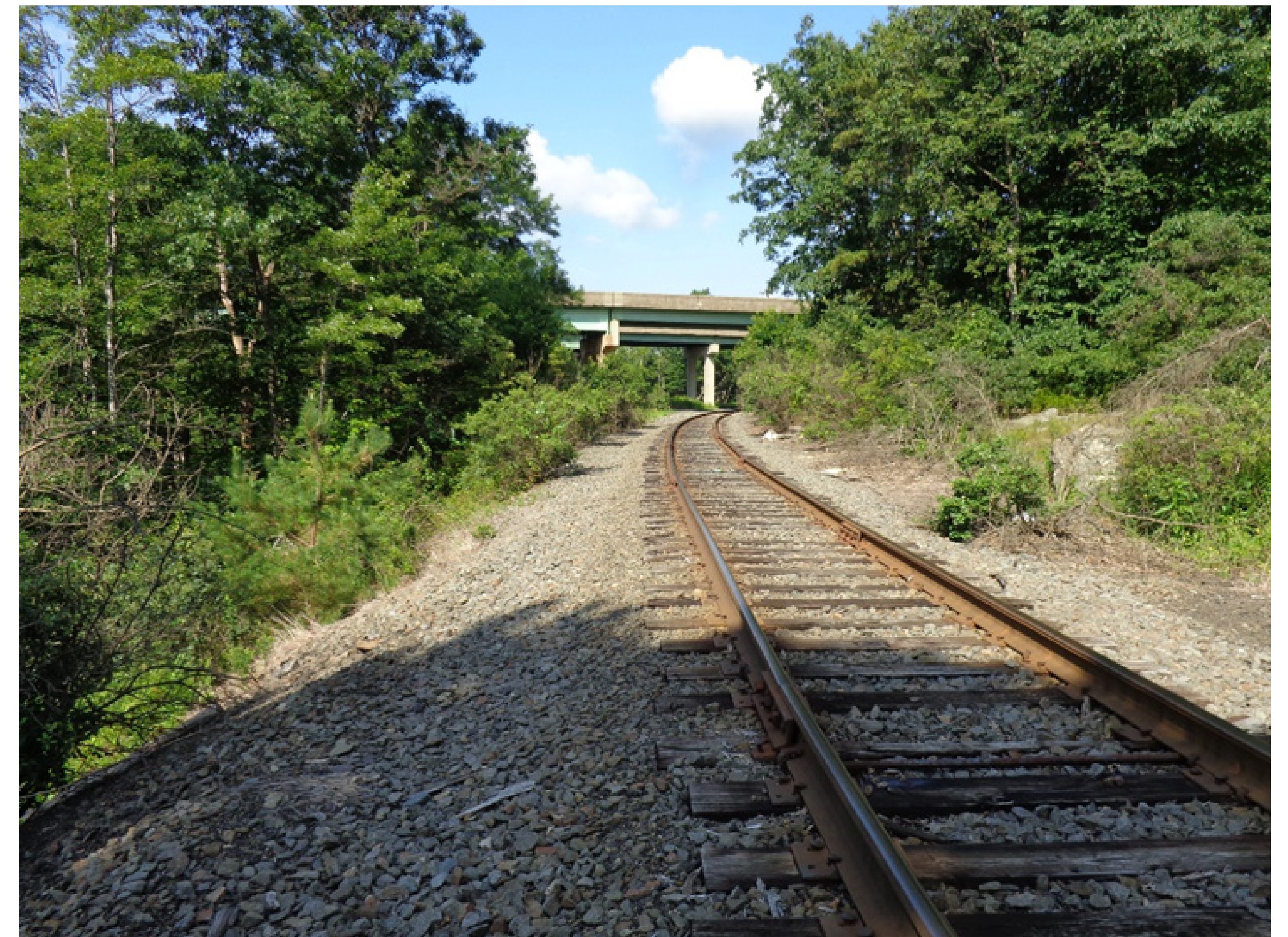
Looking west along the railroad line towards the I-81, Section 361 bridge
