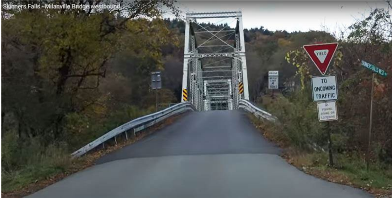
Figure 8: New York Approach geometry with a view west of the approach on the east (New York) side of the bridge.
