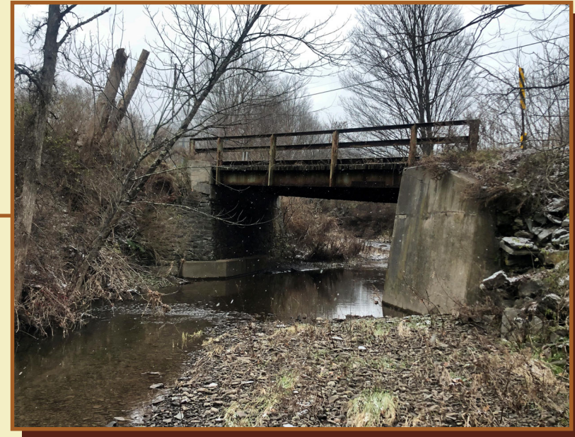
Existing Field Brook Bridge - Looking North
