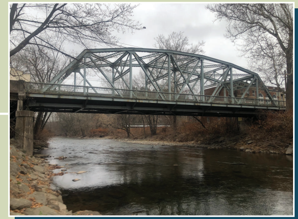
Existing Bridge Street Bridge
