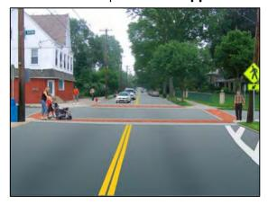
Techniques that can help improve pedestrian conditions include enhancing the visibility of the crosswalk markings with a raised or textured crosswalk. Raised crosswalks can also reduce vehicle speeds.
