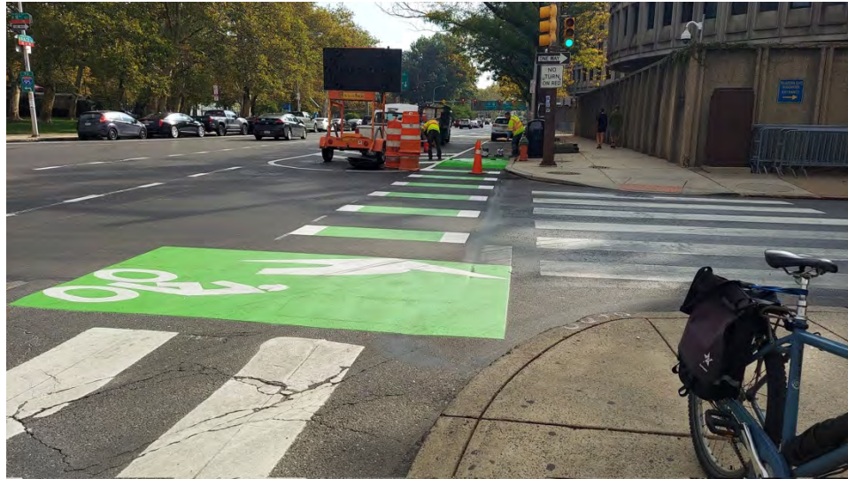
Race Street Under construction, Summer 2021
