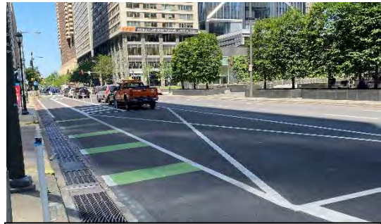
Daylighting and conflict markings at driveway on JFK
