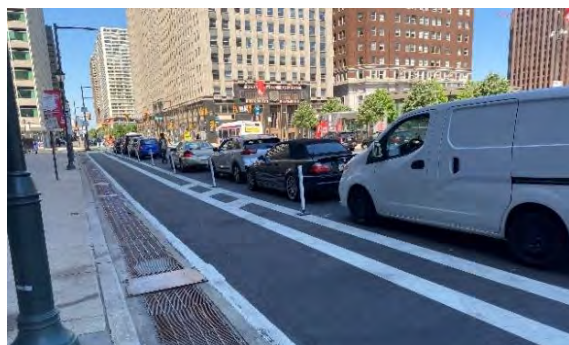
JFK Blvd PSBL mid-block location, with drainage grates and fully occupied parking
