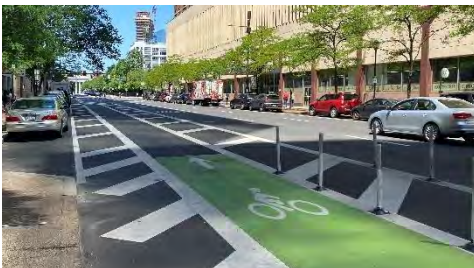
Buffered bike lane on one portion of the JFK facility
