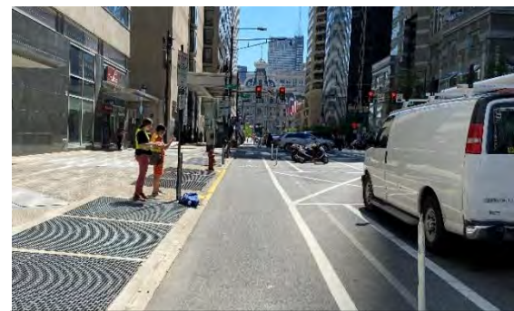
Restricted sight distance at driveway on 1700 block of Market Street
