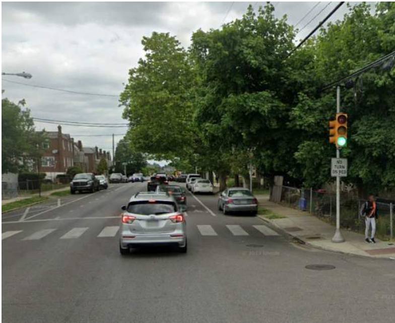
Pedestal Mounted Signal
