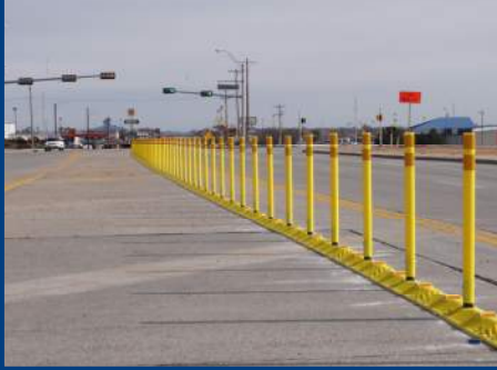
Lane Separator Curb Example
