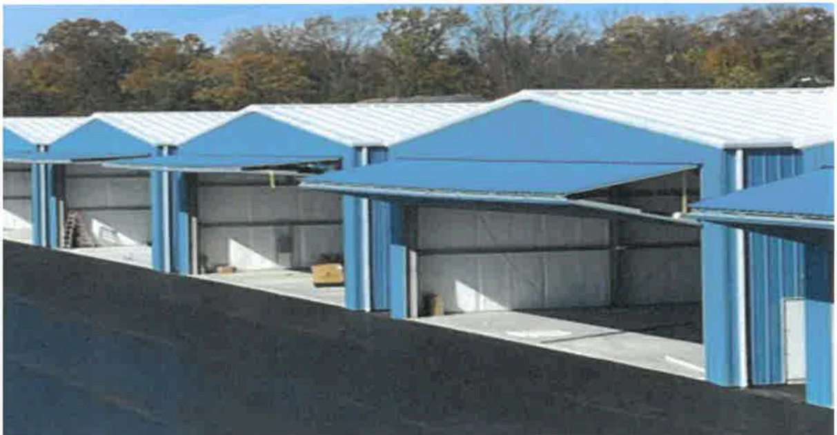
Newly Constructed Box Hangars at New Garden Flying Field Photo Courtesy of TranSystems
