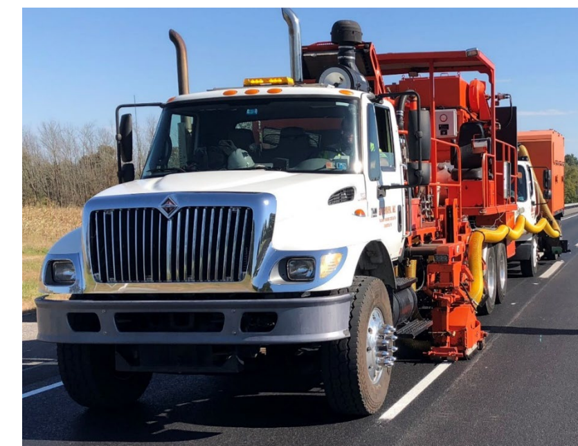
Grooving Truck Cutting Pavement Recess
