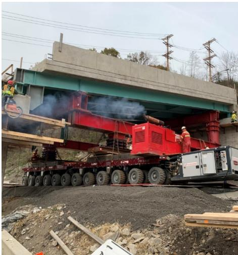
**What is it?** Self-Propelled Modular Transporters (SPMTs) are motorized vehicles that can move fully loaded at walking speed, or 3 mph, and are capable of carrying large structures, such as bridges, from offsite locations, positioning them precisely into final position. The SPMT then exits the site, opening the area to traffic possibly in minutes to within a few hours.
