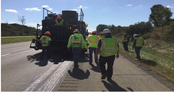
**What is it?** PennDOT District 11's Lawrence County used a microsurfacing treatment to address centerline and edgeline failures on asphalt pavement.
