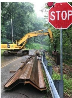
**What is it?** Sheet piles are sections of sheet materials with interlocking edges that are driven into the ground to provide earth retention and excavation support. Sheet piles is an innovative landslide repair technique used to help stabilize slopes.
